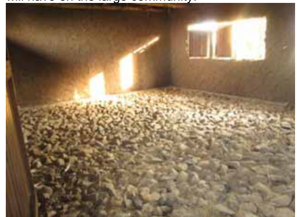
Waiting for the concrete
